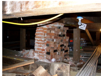
The brick foundation of fireplace/chimney at the Annie B. Ryan Field School sustained damage in the January 9 earthquake. Brick rubble to the left of the brick with mortar joints is the result of the quake's force. The unstable masonry has since been removed.
